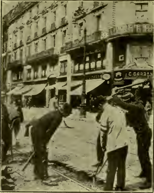
FRENCH PRISONERS REPAIRING THE TRAM LINE IN FRANKFORT.
