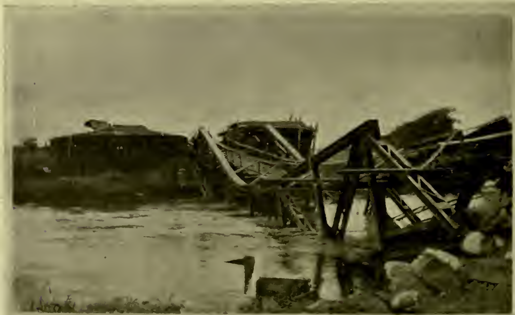
KAHE BRIDGE, PANGANI RIVER, BLOWN UP BY THE GERMANS.
