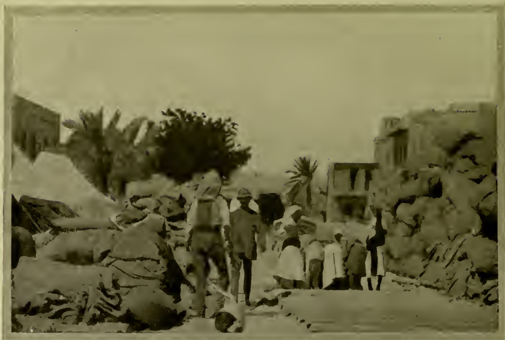
ARAB COOLIES PILING BRITISH OFFICERS' TENTS.
