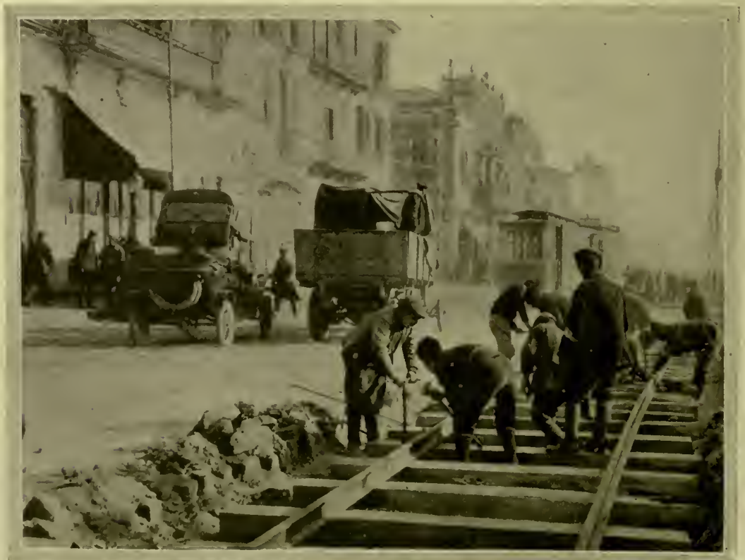
LAYING A RAILWAY THROUGH SALONIKA.
