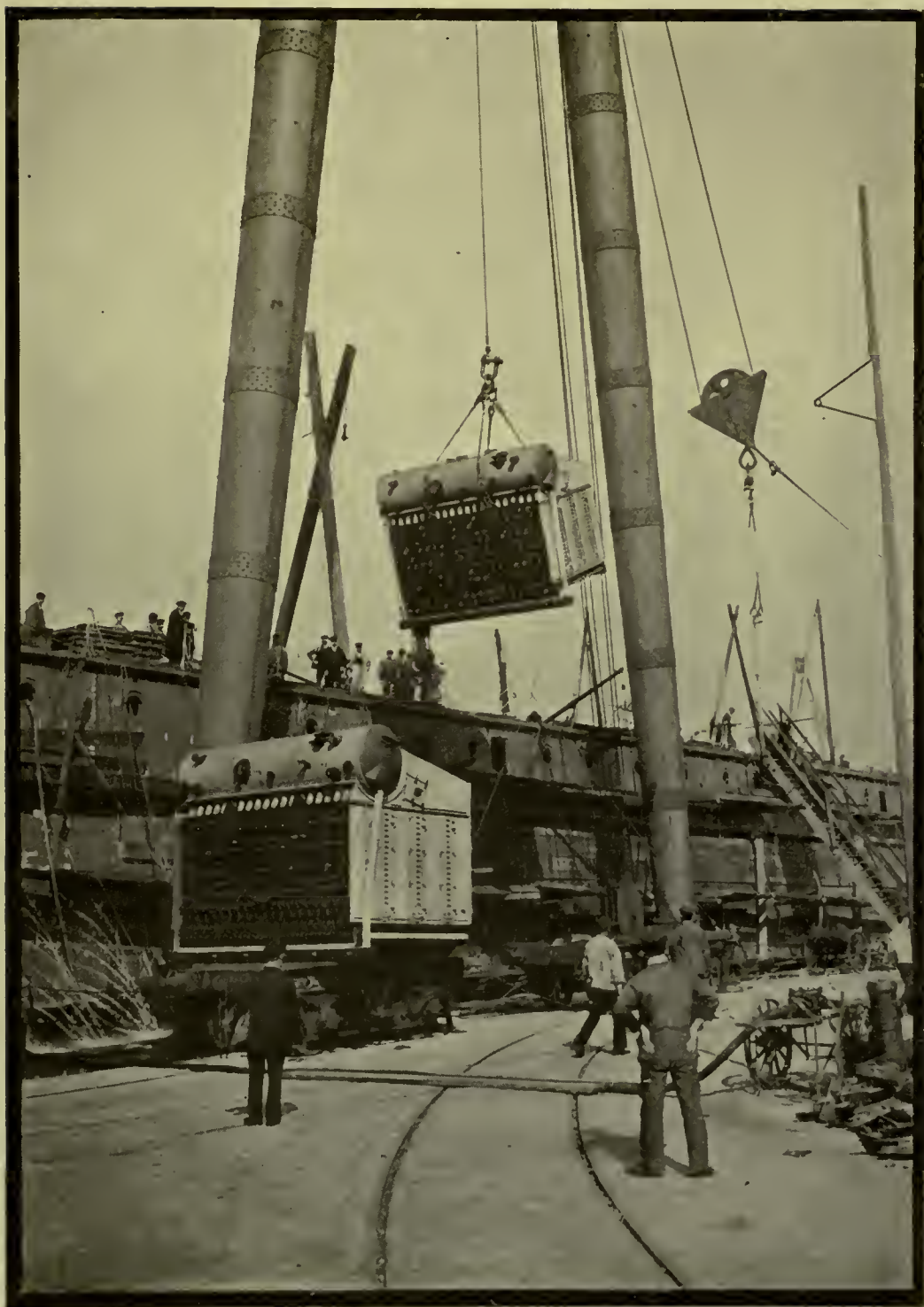
HOISTING WATER-TUBE BOILERS ON BOARD.
