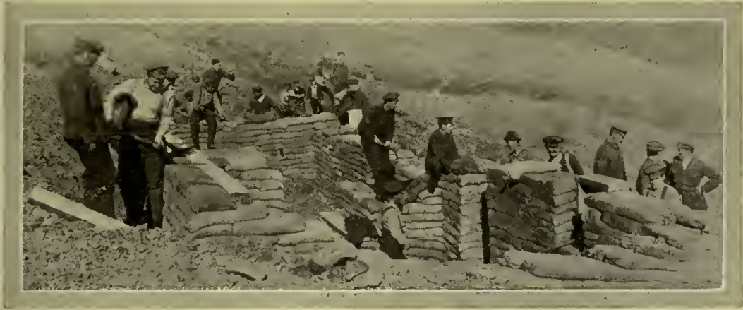
BUILDING A SANDBAG VILLA ON THE HILLS.
